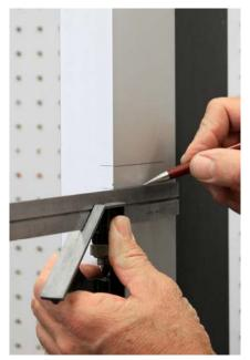
Use a combination square and transfer the lines on the front edge of the door to the side. This will show the location of the bolt when it is in the locked position.
