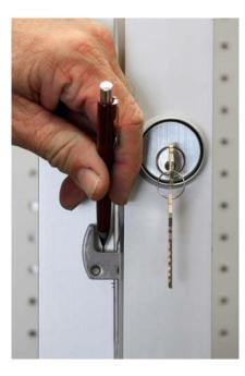
For height alignment, throw the bolt and close the door until it makes contact with the door jamb. Use a pencil and mark the top and bottom of the hook bolt. Mark the hook area of the bolt as shown.
