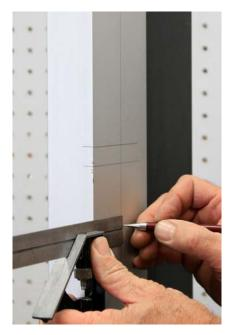
Find the center line of the jamb. This example shows the center line on a 4" wide center hung door. The center line is 2". Use a combination square and draw a vertical line at this point. Note: The center line on an offset hung door will be half the distance from the door stop to the outside of the jamb.
