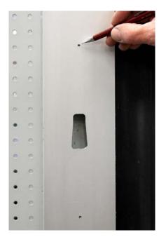
The two small template mounting holes left by the tek screws can be left as is. Or can be drilled out to 1/8" and filled with a steel pop rivet.
