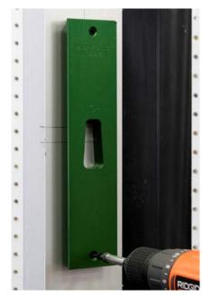
We will route the strike opening with our HIT-40AR6 template. Use the alignment marks on the template to align with the pencil lines on the jamb. Attach to jamb with the supplied tek point screws and an electric drill. Make sure the template is square to the jamb prior to running the second screw in.
