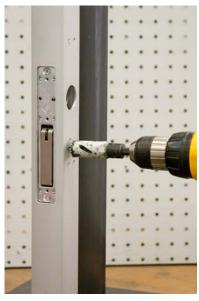
AFTER ALL HOLES 5/32" HOLES ARE DRILLED, REDRILL ONLY THE TWO INDICATOR HOLES TO 7/8" WITH A HOLE SAW. ALTERNATE DRILLING BETWEEN BOTH PILOT HOLES A LITTLE AT A TIME. DRILLING ONE HOLE THROUGH AT ONCE WILL REMOVE THE SECOND PILOT HOLE.
