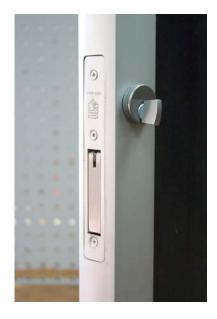
INSIDE VIEW OF ADAMS RITE DEAD BOLT LOCK. THIS HAS A STANDARD T-TURN CYLINDER TO BE REPLACED WITH A 4550 DEAD BOLT LEVER.
