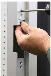
Install factory mounting tabs, leave them a little loose and tighten after the strike has been installed.
