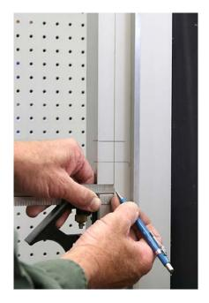
With a combination square, establish the centerline of the jamb. This is one half the distance from the door stop to the front edge of the jamb. If this distance is 1-3/4 inches, the centerline would be at 7/8 inches.
