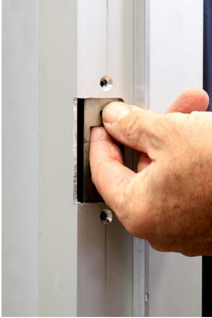
Factory mounting bracket being installed.
