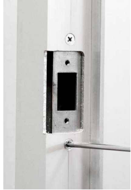
Finished installation showing strike and dust box.
