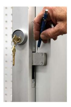
For height alignment, throw the bolt and close the door until it makes contact with the door jamb. Use a pencil and mark the top and bottom of the bolt.
