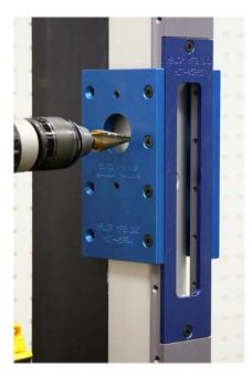
Drill the same starting holes for the lock cylinder.
