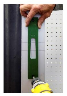
We will route the strike opening with our HIT-40AR5 template. Use the alignment marks on the template to align with the pencil lines on the jamb. Attach to jamb with the supplied tek point screws and an electric drill. Make sure the template is square to the jamb prior to running the second screw in.
