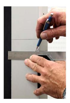
Use a combination square and transfer the lines on the front edge of the door to the side. This will show the location of the bolt when it is in the locked position.
