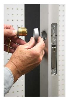
Install the outside cylinder. We recommend the addition of one of our hardened cylinder guards for security.
