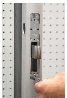
Secure lock with the screws supplied with the mounting bracket.
