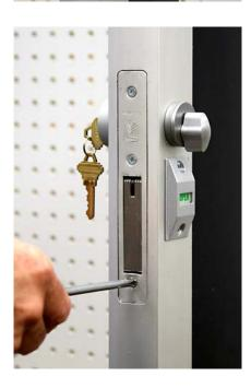
Install the faceplate and the lock is installed.
