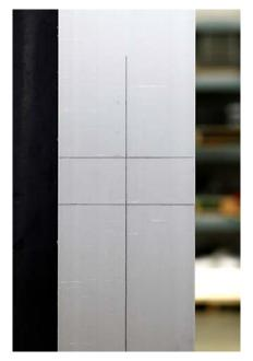
Pencil lines showing the center line of the jamb and the height of the bolt when in the locked position have now been established.
