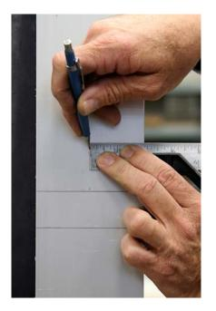
Find the center line of the jamb. This example shows the center line on a 4" wide center hung door. The center line is 2". Use a combination square and draw a vertical line at this point. Note: The center line on an offset hung door will be half the distance from the door stop to the outside edge of the jamb.
