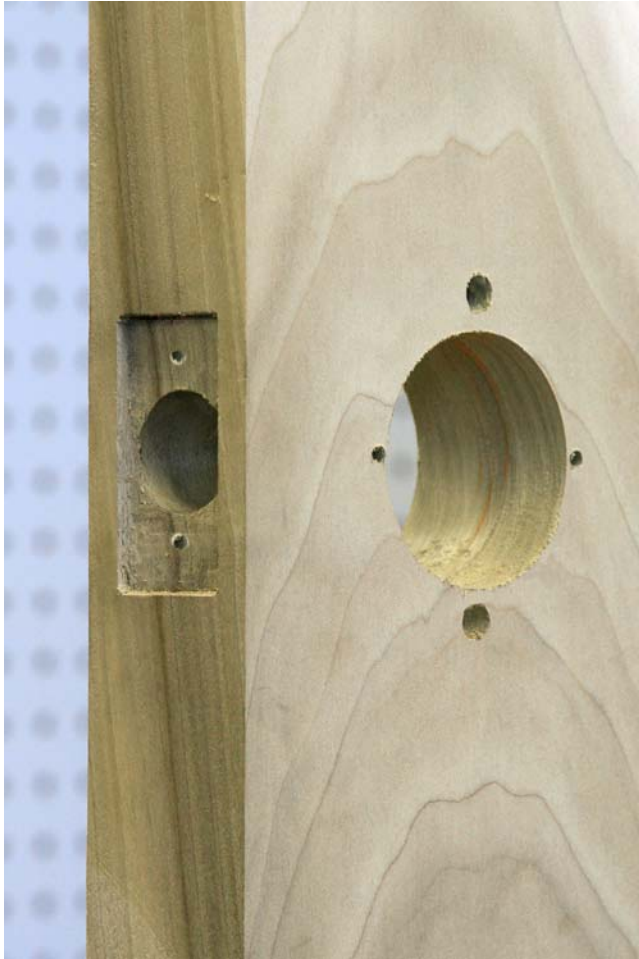
Completed lock prep.
