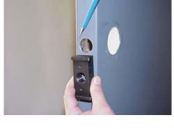
Center the forming die over the latch hole. Pencil mark on door edge shows center of latch hole, the forming die has an alignment mark to locate the center of the die. Make sure set screws in form die are backed off inside die. They must not protrude at this time.
