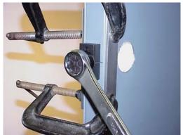
Use the supplied hex key and tighten the top and bottom set screws in the forming die. This will locate the latch mounting screws.
