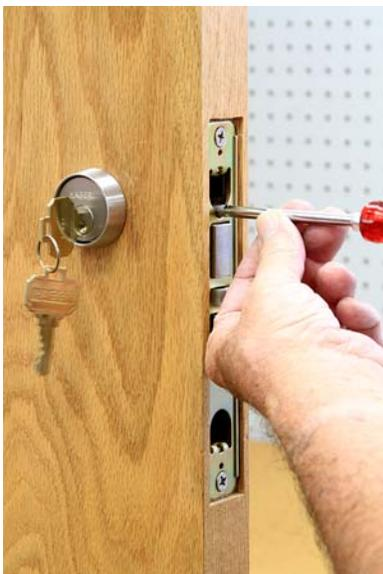
Tighten the mortise cylinder retaining screws and install the faceplate.
