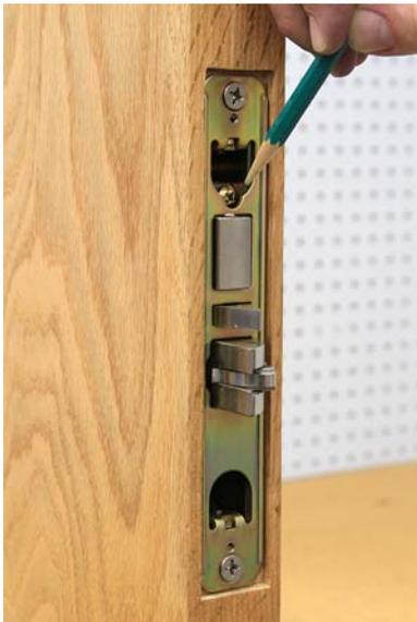
You need to locate the approximate location of the cylinder hole and can do so as follows: Using the cylinder retaining screw as a center point draw a line with a combination square. This is the horizontal center line of the cylinder.
