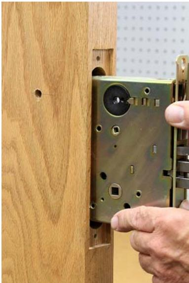
Install the lock case back into the door.
