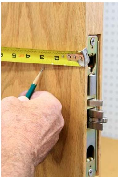
Measure backset of the lock, in this case 2-3/4" and make a second mark. This is the approximate center of the cylinder hole.
