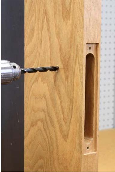
Drill a 3/8" to 1/2" hole at the marked location this should be close to the center of the cylinder hole.
