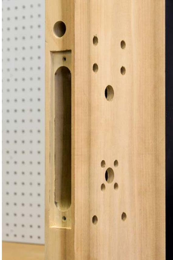
When all holes have been completed remove the HIT-66 system and alignment fixture from the door.
