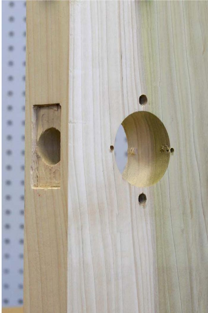
Remove HIT-111 from door and install cylindrical lever per manufacturers directions.
