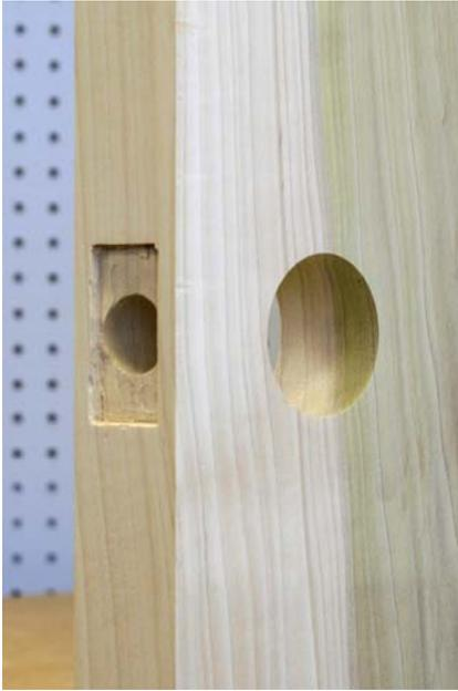
With the use of the HIT-111, a standard 2-1/8" door prep can easily and accurately be retrofitted to accept a number of different cylindrical lever handle locks.
