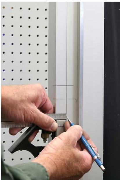
With a combination square, establish the centerline of the strike. The door and strike need to have the same center line. For a standard 1-3/4" door this dimension is 7/8" from the door stop if the lock is centered in the door channel. If the lock is off center, adjust accordingly. The face of the electric strike and the face of the lock must be centered together when the door is closed.
