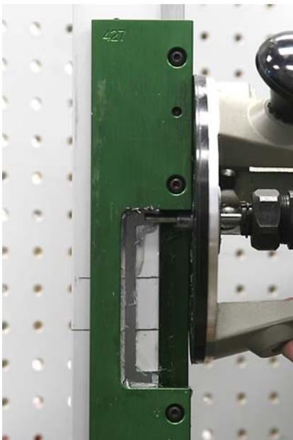
Place the router at the top of the template, you will be routing the faceplate area. The router guide should be touching the electric strike template with the bit not making contact with the frame. Let the router come to full speed and route through the side of the jamb. Be sure to hold the router flat against the template and **DO NOT BACK UP IN THE CUT**. When completed at the top, **LET THE ROUTER COME TO A COMPLETE STOP BEFORE REMOVING IT FROM THE TEMPLATE**
