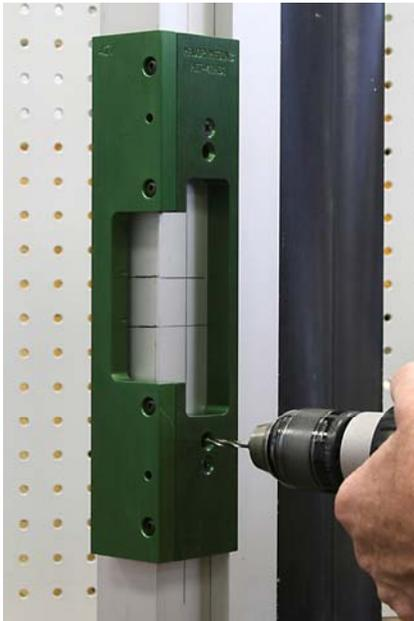
Some HIT-41 templates have one screw hole top and bottom and some have two. These holes will align the factory mounting tabs needed later, some factory tabs are mounted with one and some with two. How many are needed depends on the strike you are using. One screw top and bottom will hold the template. The second hole for the tab can be located by drilling with a 9/64" drill bit or by using a second screw.
