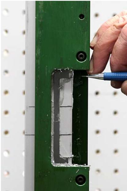
Note that we did not route through the top of the lip area, this will be cut out with the next pass. If you run through the side wall you run the risk of hitting the template with the router bit.
