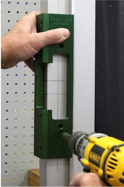
Align the HIT-41 template to the pencil marks and attach to the jamb using tek point dry wall screws. It is a good idea to use a drill with a clutch feature, you don't want to snap the screw off in the jamb.
