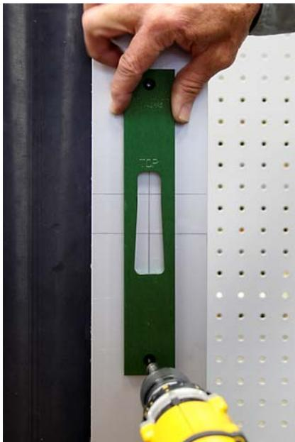
We will route the strike opening with our HIT-40AR5 template. Use the alignment marks on the template to align with the pencil lines on the jamb. Attach to jamb with the supplied tek point screws and an electric drill. Make sure the template is square to the jamb prior to running the second screw in.
