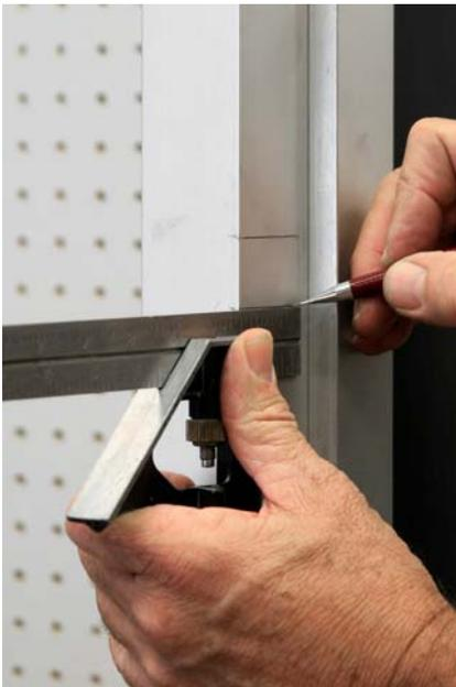
Use a combination square and transfer the lines on the front edge of the door to the side. This will show the location of the latch when it is in the locked position.
