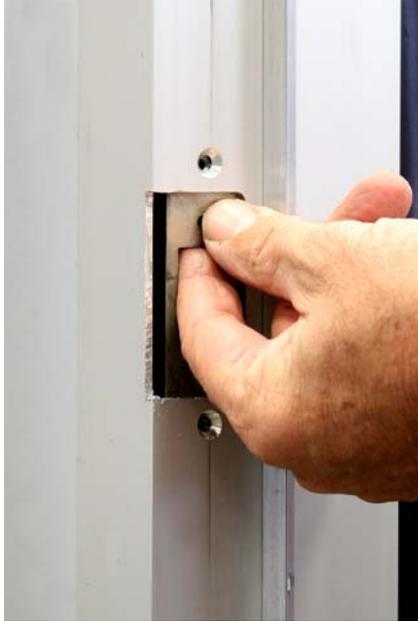
Factory mounting bracket being installed.
