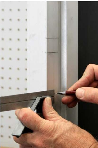
Find the center line of the jamb. This example shows the center line on a 4" wide offset hung door. The center line is  $\frac{7}{8}$ " from the stop, or one half the thickness of the door. Use a combination square and draw a vertical line at this point.
