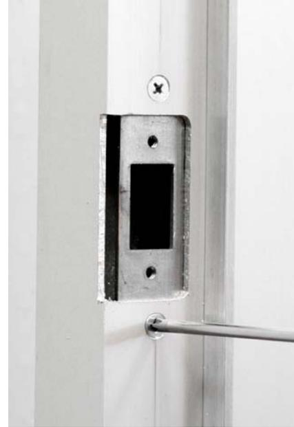
Finished installation showing strike and dust box.
