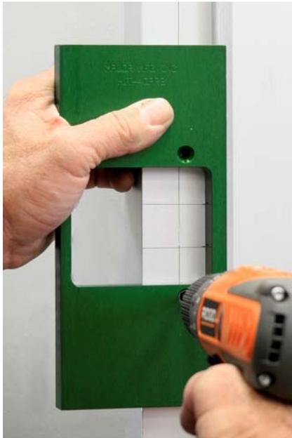
Pencil lines showing the center line of the jamb and the height of the bolt when locked have been established. Use the alignment marks on the template to align with the pencil lines on the jamb. We will route the strike opening with our HIT-40AR3 template. Attach to jamb with the supplied tek point screws and an electric drill. NOTE: It is a good idea that your drill is equipped with a clutch feature, this will prevent snapping the screw off in the jamb.
