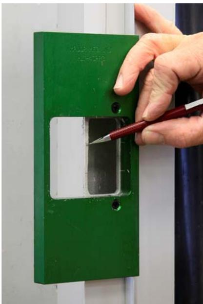
This is the area you did not cut through in the step above. Adjust the depth of the router to cut the thickness of the jamb material only, this should be a cut depth of only about 1/8 inch. Use the router to nibble away this area.
