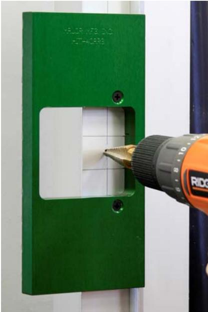
Drill a 3/8" or larger starting hole for the router bit in the center of the template hole to be routed. In the picture we are using a step drill bit.
