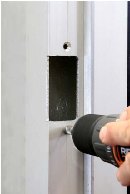
Counter sink both holes for the 10-32 flat head mounting screws supplied by the factory.
