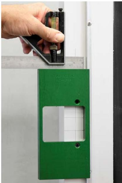
Make sure the template is square to the jamb prior to running the second screw in.
