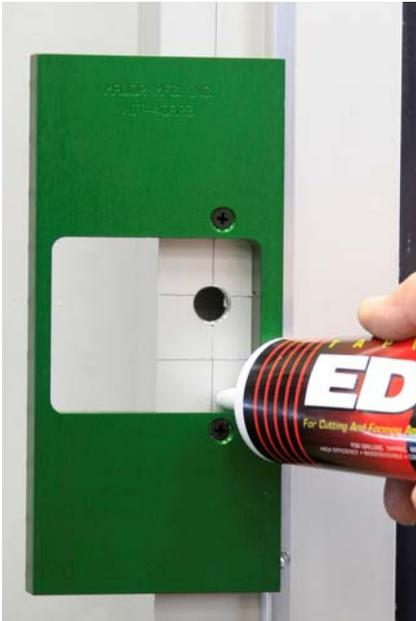
We recommend the area to be routed be lubricated with a cutting lube. We use a product called Tapmatic Edge Cream made by the LPS Company. You can find this product at industrial hardware stores or machine shop supplies. This is also a handy product to use for other drilling or tapping chores.
