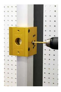
Change to a 7/32" bit and drill the right and left hand rim cylinder screw holes.
