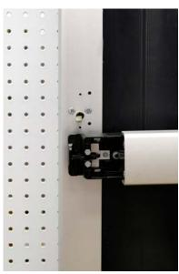
Finish installing panic hardware and strike per Adams Rite directions. There are two 5/32" holes required on the opposite side of the panic bar. Simply level bar to the door and drill through the holes in the bracket for alignment and install mounting screws.
