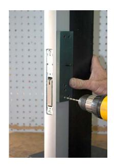
DRILL ALL HOLES WITH A 5/32" DRILL BIT. INSERTING A SECOND 5/32" BIT BACKWARDS INTO THE FIRST HOLE DRILLED WILL LOCK THE TEMPLATE IN POSITION.
