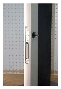
HIT-22 ALIGNMENT GUIDE INSTALLED AND ALIGNMENT PIN INSERTED IN HOLE.
