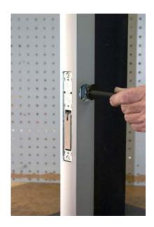
HIT-22 ALIGNMENT GUIDE ABOUT TO BE INSTALLED IN CYLINDER OPENING. TIGHTEN CYLINDER SET SCREW AND REMOVE INSTALLATION HANDLE.
