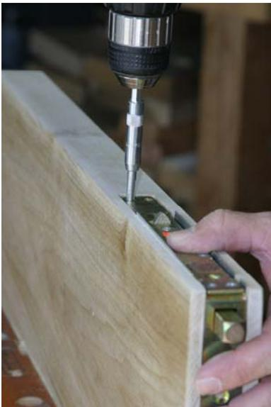
Use a center drill and drill screw mounting holes and install flush bolt per manufacturers instructions.
