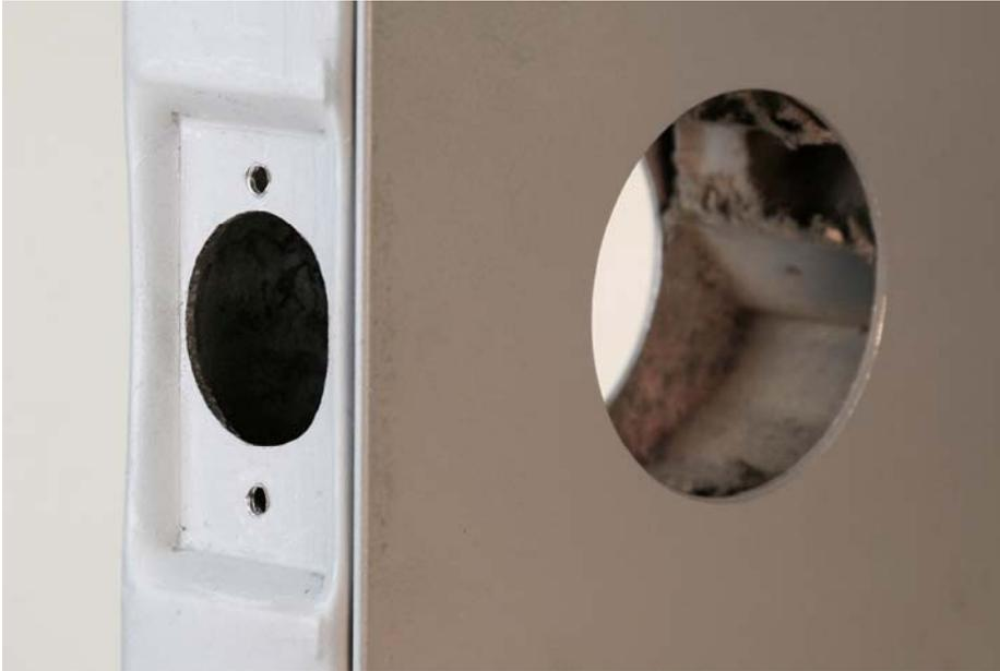
Lock prep with faceplate indentation made by our Pit Bull tool. The HIT-24 will also work if you use a cut out and mounting brackets.
