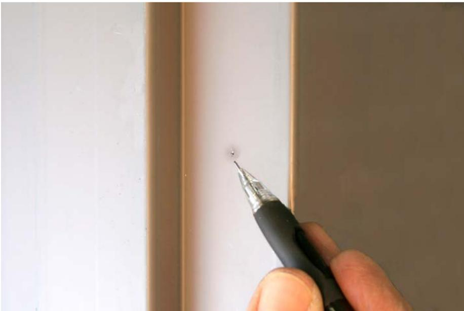
This is the exact center of the strike. Use this point to establish layout lines required for the strike cutout. See a listing of the strike mounting brackets we offer on our web site to mount strikes plates in steel jambs.
