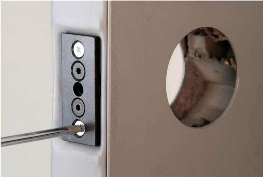
HIT-24 guide being mounted in door. Use the mounting screws supplied with the lock being installed to hold in place.
