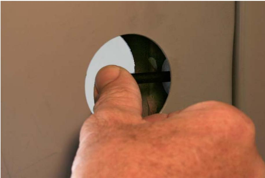
Apply pressure to the locator point to leave a mark on the door jamb.
