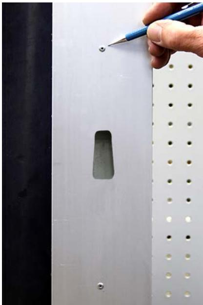
Finished installation showing mounting holes filled with a pop rivet.
