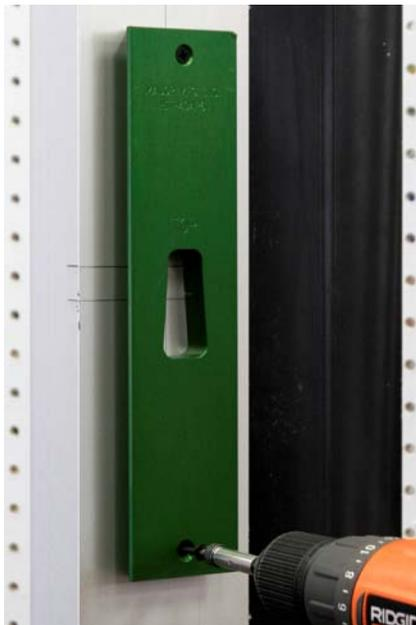
We will route the strike opening with our HIT-40AR6 template. Use the alignment marks on the template to align with the pencil lines on the jamb. Attach to jamb with the supplied tek point screws and an electric drill. Make sure the template is square to the jamb prior to running the second screw in.
