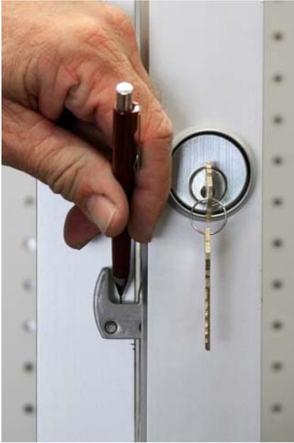
For height alignment, throw the bolt and close the door until it makes contact with the door jamb. Use a pencil and mark the top and bottom of the hook bolt. Mark the hook area of the bolt as shown.
