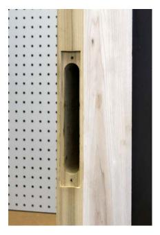
Shown is a standard mortise pocket, we will use this as a basis for the Sargent Mortise Lock install.
