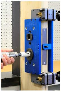
With a 1-1/8" hole saw drill the lock spindle hole. Drill both sides of the door to the mortise pocket.
