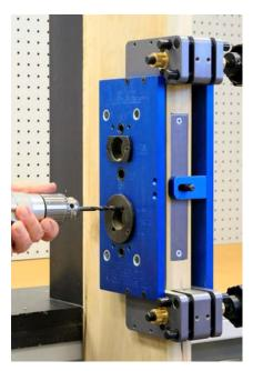
Drill the thru-bolt holes with a 1/4" drill. Drill from both sides of the door to the mortise pocket.
