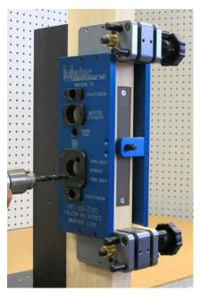
With a 3/8" twist drill, drill the thru bolt holes on both sides of the door. These holes go to the mortise cavity. Do not try to drill from one side through to the other.
