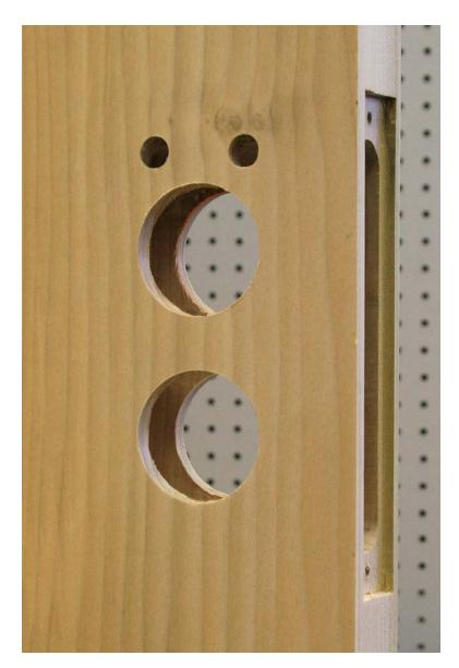
Completed lock prep. Install lock per manufacturers directions.
