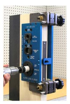
Change to a 1-1/4" hole saw and drill the lever hole. This hole goes to the mortise pocket from both sides of the door.
