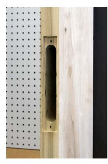
Shown is a standard mortise pocket, we will use this as a basis for the Alarm Lock Installation.
