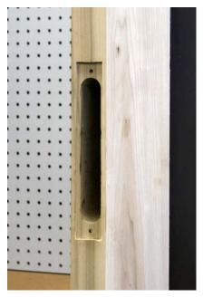
Shown is a standard mortise pocket, we will use this as a basis for the Marks Mortise Lock install. While a new install is shown, this drill guide is the perfect tool for a retrofit install.
