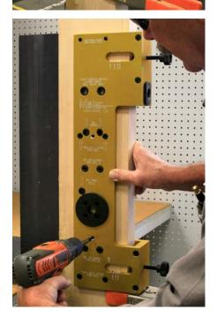
Attach the guide to the door with 2 of the supplied #6 dry wall screws. The attaching holes are counter sunk and are on both sides of the door. **MOUNT THESE SCREWS ON THE INSIDE ONLY**. Use a drill with a clutch system so you don't snap the screws off when they bottom out in the countersink. The screw holes will be covered by the head of the device after it is installed, they will not be visible.
