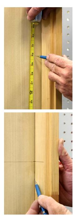
Locate the horizontal center line of the door and draw a locating line. This will be the center line of the device. According to Von Duprin this will be 39-13/16" to the **finished floor**. Install factory strike on the jamb side aligned on this center line.
