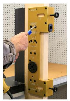
If using a door position switch, two holes will be needed on the **INSIDE OF THE DOOR ONLY.** Using the drill bushings marked door position switch, drill two 1/2" holes to a depth of 1-1/4". We used blue painters tape as a stop gauge, **DO NOT DRILL THRU THE DOOR.**
