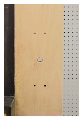
After removing an existing 99 rim device the mounting holes can be used to align the HIT-32-380 drill guide.
