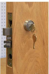
Install the outside and inside cylinders and replace the lock faceplate.
