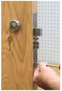
First remove the lock faceplate and loosen the cylinder retaining screw.
