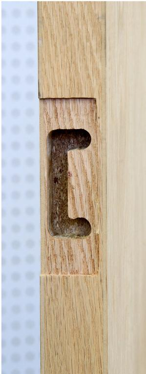
McKinney PoE (Power Over Ethernet) electrified hinge uses the U-Shaped wiring pocket as shown in our installation.
