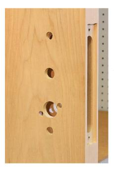
Completed installation using thru bolted trim. If using surface mounted trim see next step
