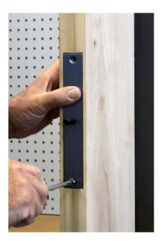
Install the mortise lock positioning plate. The plate will fit into the 1-1/4" x 8" faceplate cut out. There will be a 3/8" diameter pin centered on the plate. There is no top or bottom to worry about.
