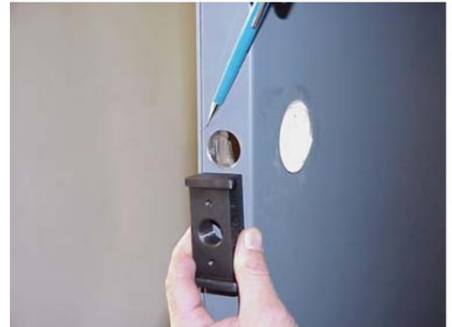
Draw die being placed inside door. Use care with this step, don’t drop die inside door. There is a 8-32 tapped hole on the back of the draw die - use to attach a wire or lanyard for peace of mind. (not supplied) Lube the threads of the draw bolt with bearing grease prior to installing the Pit Bull fixture in door. Failure to properly lube bolt may damage the Pit Bull tool.
