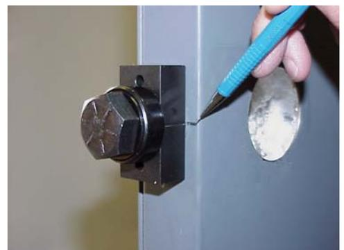
The use of the two steel bars ( supplied) and C clamps ( not supplied ) will help prevent door distortion when forming latch pocket. Clamp one on the inside and outside edge of door as shown.
