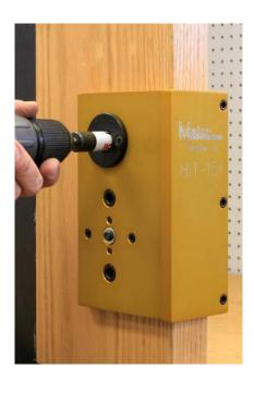
The last hole that is needed is the 3/4" through hole. In the picture we are using a hole saw. Be sure to use a slow speed and back the hole saw out from time to time to clear saw dust. You can use a twist drill on both wood or steel doors or a brad point bit on wood doors only.
