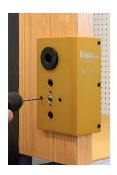
The lock you are installing uses anchor plate lugs, they can be installed by drilling two 5/32" holes using the bushings at 3:00 and 9:00 on both sides of the door. Drill to about 1/4" depth. You may need to notch these holes with a file on a steel door.
