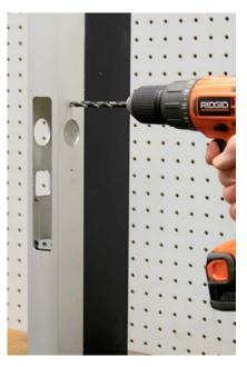
Remove the lock from the door and enlarge the two holes to 17/64" with the use of a twist drill.
