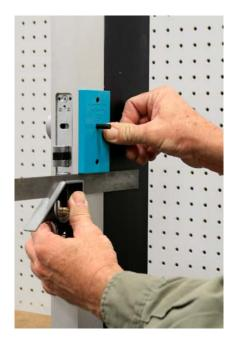
Put the 1/4" dowel pin in the HIT-22 guide and slide the HIT-40AR8 drill guide over the top. Square to the door with a combination square.
