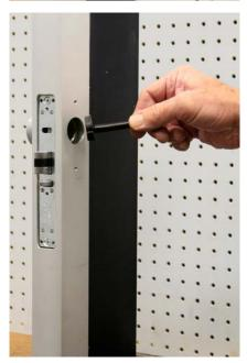
Take a second #21 drill bit and put the reverse end of the bit in the drilled hole. This will keep the guide in alignment when drilling the second hole.
