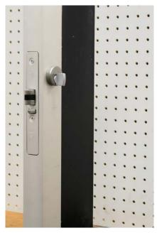
Dead latch lock with inside thumb turn cylinder.
