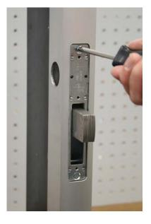
Secure lock in door using screws supplied with brackets. Installation is complete. Add lock cylinders and faceplate.
