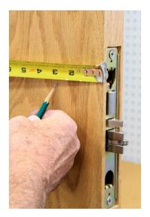
Measure backset of the lock, in this case 2-3/4" and make a second mark. This is the approximate center of the cylinder hole.
