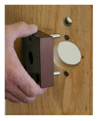
Install the wire run guide over the cross bore using the two alignment pins. Bolt to the backplate with the 3/8" allen bolt. Mount this guide on the battery side of the door.
