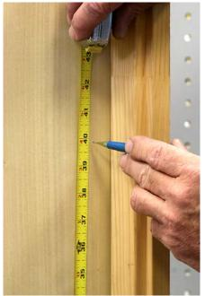
Locate the horizontal center line of the door. According to Von Duprin this will be 39-13/16" to the **finished floor**. Install factory strike on the jamb side aligned on this center line.
