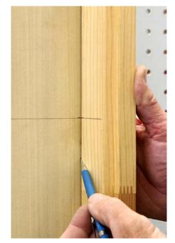
To determine the backset, draw a vertical line along the door stop onto the door.
