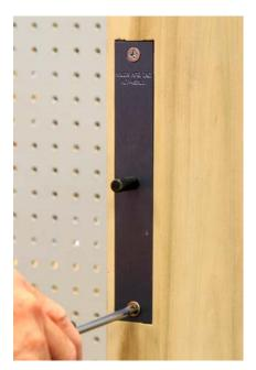
Install the mortise lock positioning plate. The plate will fit into the 1-1/4" x 8" faceplate cut out. There will be a 3/8" diameter pin centered on the plate. There is no top or bottom to worry about.
