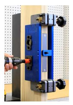
Drill to the mortise pocket from both sides of the door. Back the hole saw out once or twice when drilling to clear the chips from the cut.
