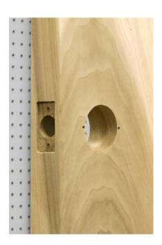
With the use of the HIT-146N, a standard 2-1/8" door prep can easily and accurately be retrofitted to accept the Schlage CO lock in just a few minutes.
