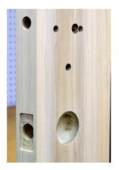
Remove the HIT-146 from the door and install the Schlage CO lock per the manufacturers directions.
