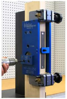
Drill 1/4" holes on both sides of the door. They will go to the mortise pocket. Do not try to drill all the way through both sides at once.
