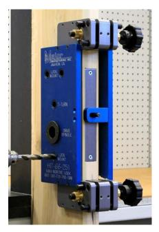
Drill the four 1/2" diameter holes on the drill guide. The two top holes and the bottom hole are lock mounting holes for thru-bolt mounting. The center 1/2" hole is for the t-turn. Drill half way from both sides of the door.
