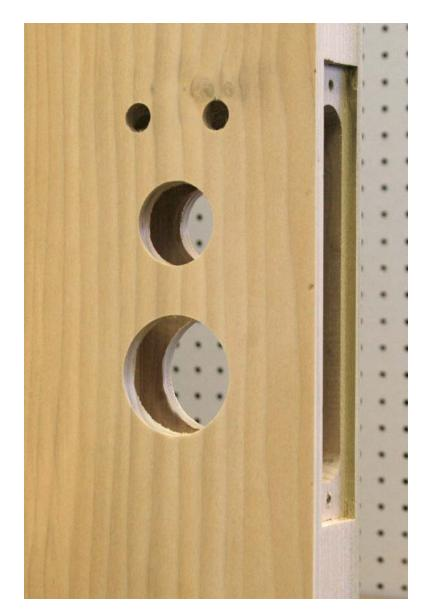
Completed lock prep. Install lock per manufacturers directions.
