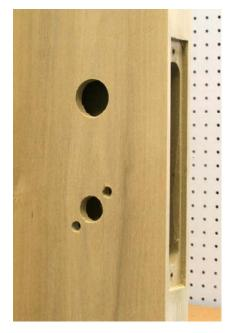
When all holes have been drilled, remove the HIT-66 drill guide from the door. This is a prep for a Best mortise lock with rose trim. If installing escutcheon trim see next page.
