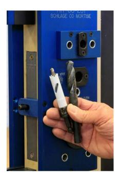
When drilling the wire run hole in a steel door, use a twist drill or hole saw as shown at left.
