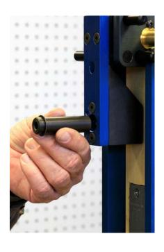
If installing in a **steel door**, do not attempt to drill this hole with a hole saw. The hole will be too big and the door position switch will not be held firmly. Install the 5/16" supplied bushing and screw.
