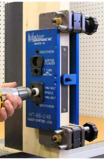
Use a 1" hole saw to drill the spindle hole. Drill this hole to the mortise pocket from both sides of the door. When drilling back the hole saw out a few times to clear saw dust from the cut.
