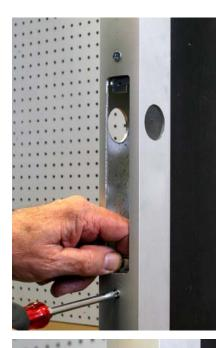
Install the bracket, do not tighten the screw all the way down at this time.
