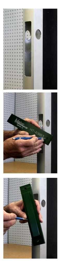
Here is a standard cut out for an aluminum door that will accept an Adams Rite style Lock. The cut out will be the same for a swing bolt, hook bolt or deadlatch. It will also be the same for a deeper style lock.
