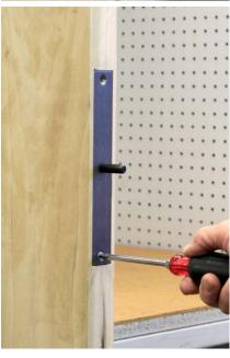
Last, install the two mortise lock screws to hold the plate during the install. This will also make the lock body easier to install when completed.
