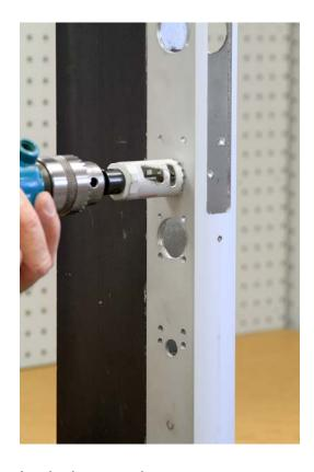
Use a 1-1/8" hole saw and drill the two exterior holes as shown.
