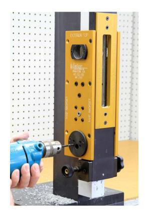
With the same 3/16" bit in the drill, drill the remaining holes on the exterior template. There are five holes on the template and two on the large drill bushing. Two holes on this side are pilot holes and will be drilled out after the clamp and template are removed from the door.
