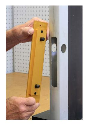
If this installation is new, a faceplate will need to be cut in the door, attach a HIT-30AR11 to the clamp. (LH picture) If you are retrofitting an existing door prep, attach a HIT-30AR20 alignment guide to the clamp. (RH picture)
