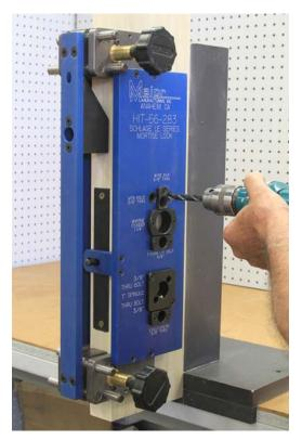
Upper mounting holes being drilled with a 3/8" twist drill bit. Be sure to drill half way from both sides of the door.
